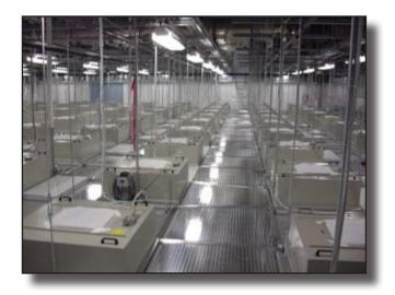
Fan Filter Units are typically used in place of conventional recirculating air units due to height restrictions and are often installed in a ceiling grid system or suspended from a support structure. Recirculated air is purified through a prefilter installed on the top and blown through a HEPA or ULPA filter into a cleanroom.
