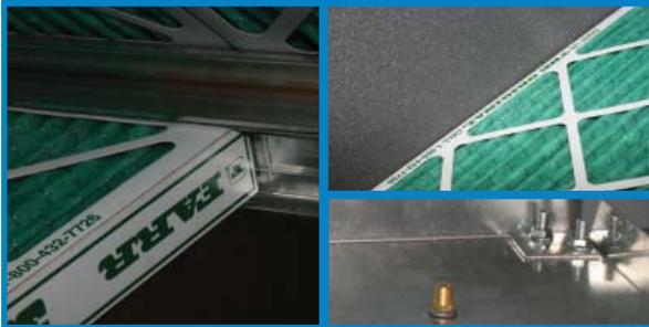
*Left:* Filters are sealed into place by a fin seal on the filter track that eliminates air bypass and ensures cleaning of all air through the housing.
